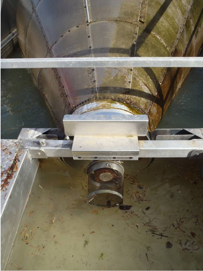
Photo of Cone Guard and Shaft Guard (modified minnow trap).
